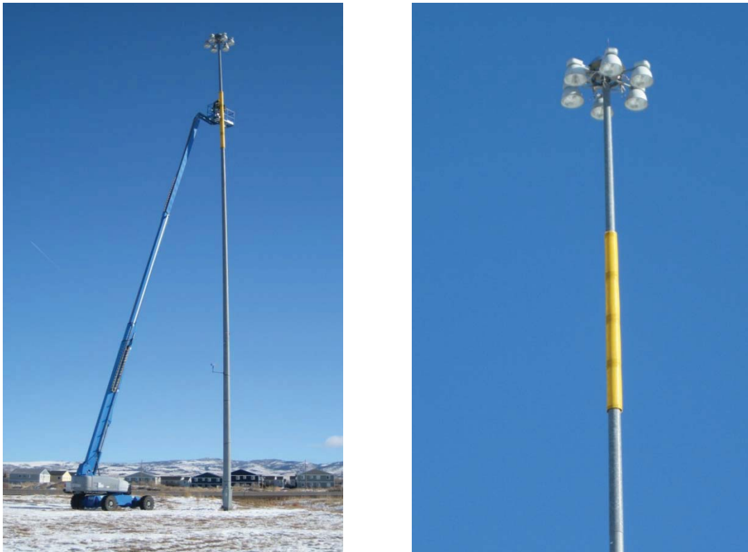
Figure 52. Perforated shroud installed on high-mast pole
