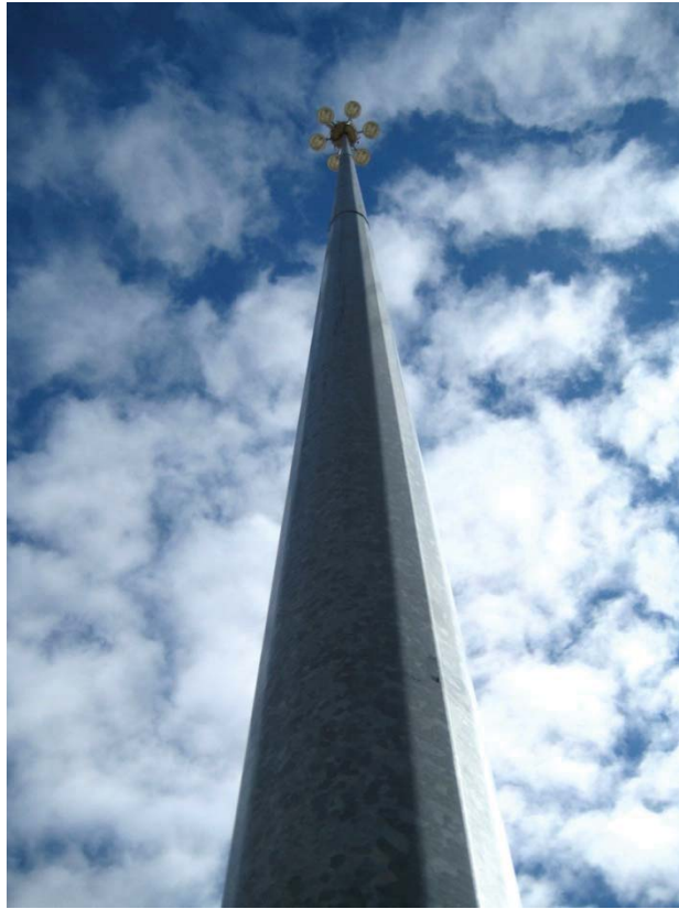
Figure 1. 120-ft, 16-sided high-mast light pole
