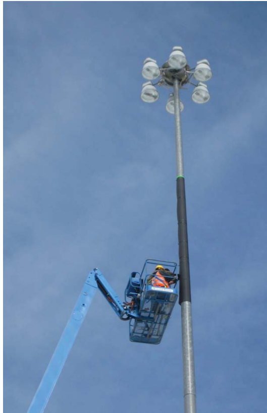
Figure 55. Surface roughness installed on high-mast pole
