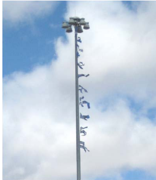
Figure 50. Ribbon retrofit on top 40 ft of high-mast pole
