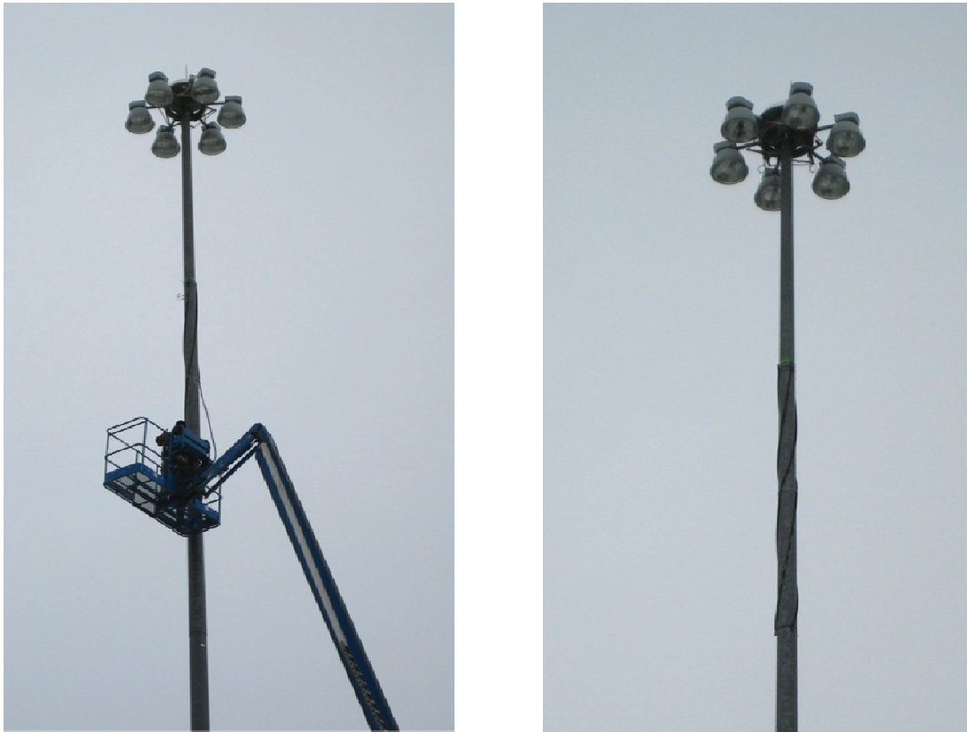
Figure 51. Helical strakes installed on high-mast pole
